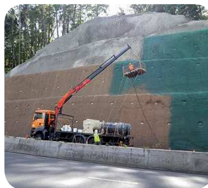
Hydroseeding application (Euro-Tec, France)
